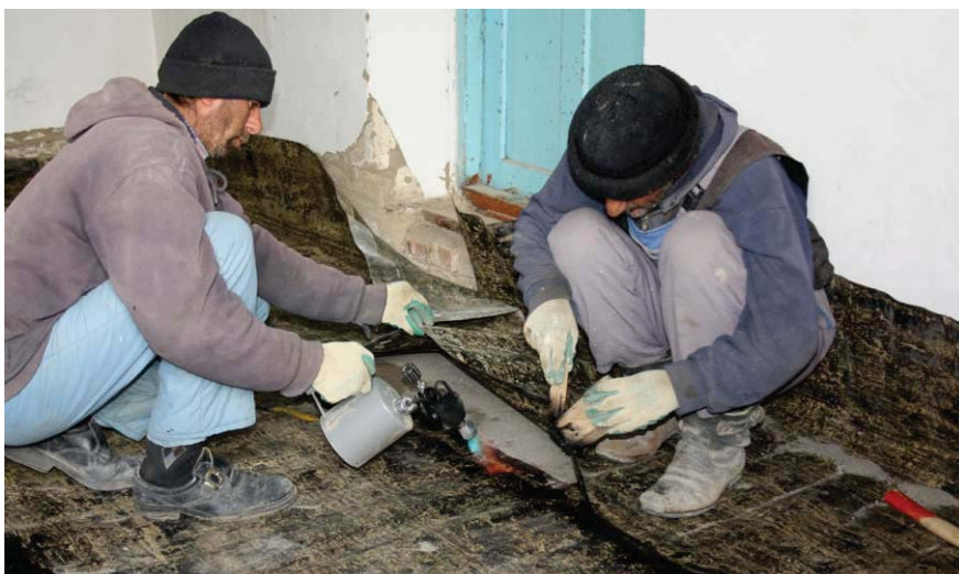
A team of two construction workers is working on the insulation of the floor in a house in the town of Murgab, Gorno-Badakhshan.
