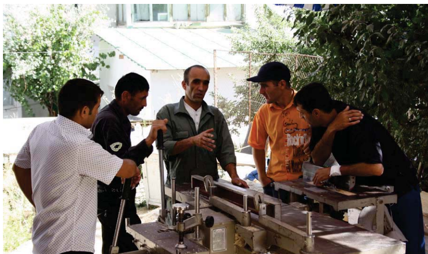
Local carpenters are trained in producing well-insulated wooden doors and windows in the town of Khorog, Gorno-Badakhshan.
