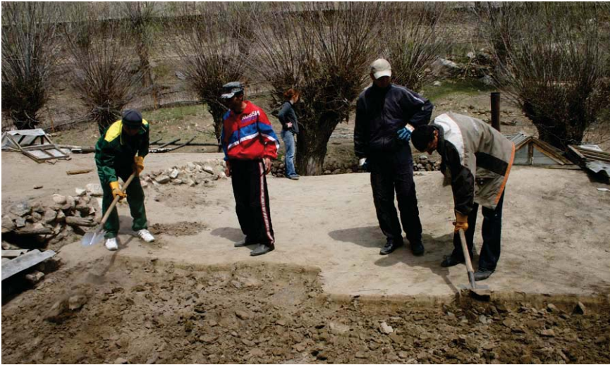
Construction workers are working on the insulation of a roof in a village in Gorno-Badakhshan.
