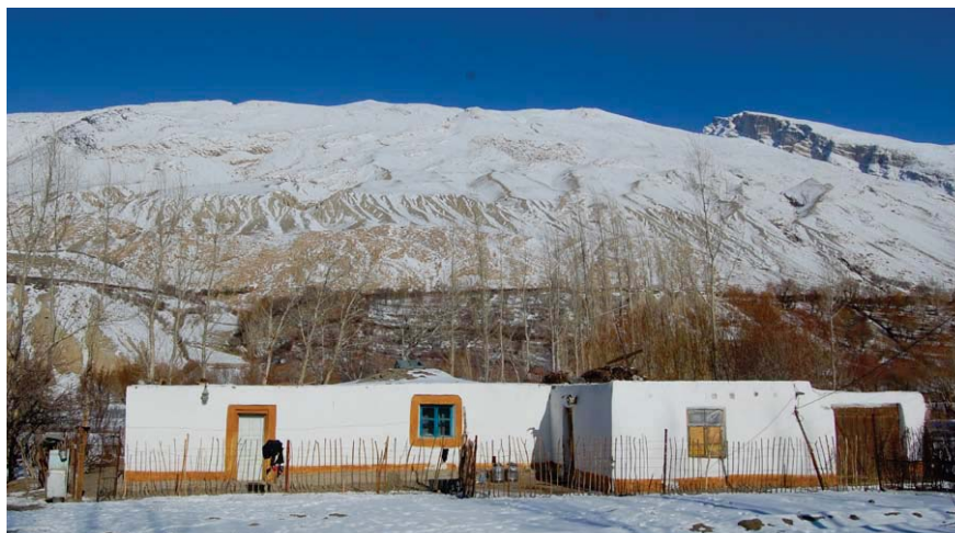
A house in the village of Langar in Gorno-Badakhshan, at an elevation of almost 3,000 meters above sea level. Winters here are long and cold, and firewood is not cheap, therefore thermal insulation is an attractive option for the villagers.
