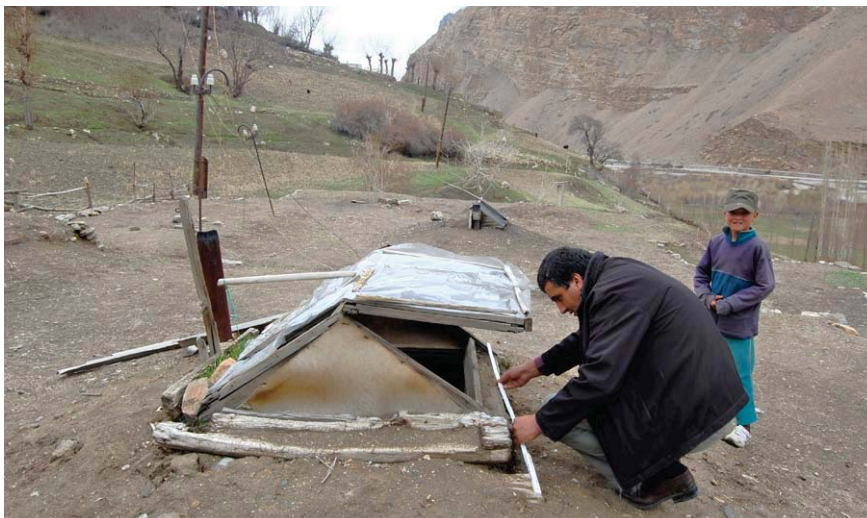
On a house in the village of Barvoz in Gorno-Badakhshan, the old roofhatch-window is measured in order to determine if the size of the new one will fit well.
