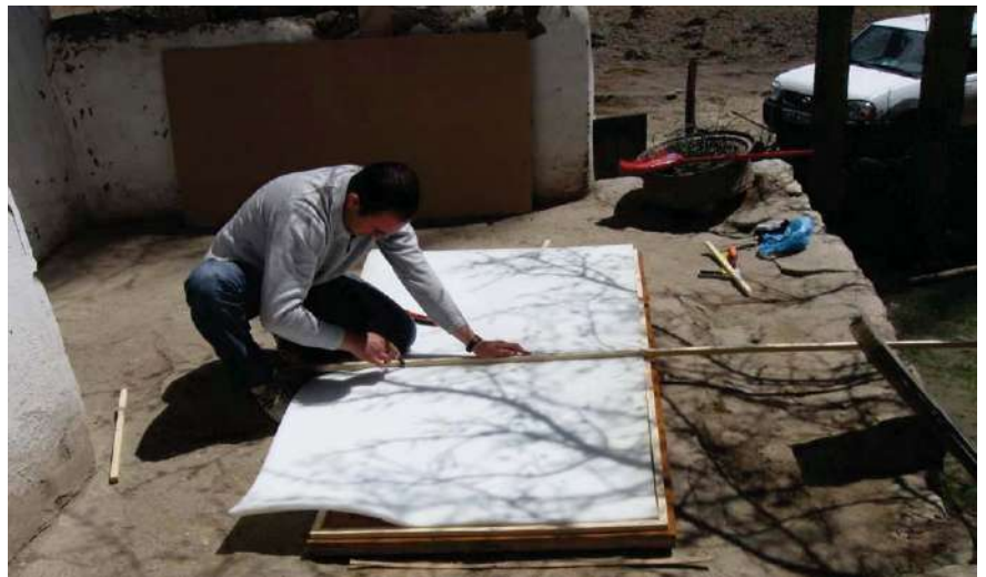
An old door is covered with insulation material in a village in Gorno-Badakhshan. In some cases, this is a viable alternative to the installation of a new door.
