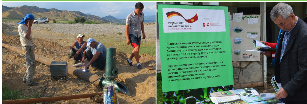
Installation of hydraulic ram pumps in Kyrgoo village of Bazar-Korgon district, Kyrgyzstan.
